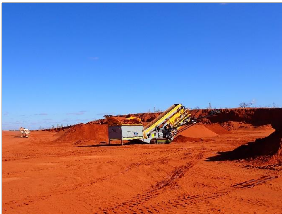
Plate 2-3 Example of Screening Plant within Excavation Area
