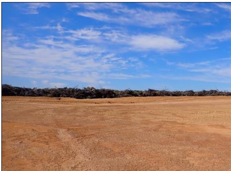
Plate 2-2 Example of Vegetation Stockpile Along Excavation Area
