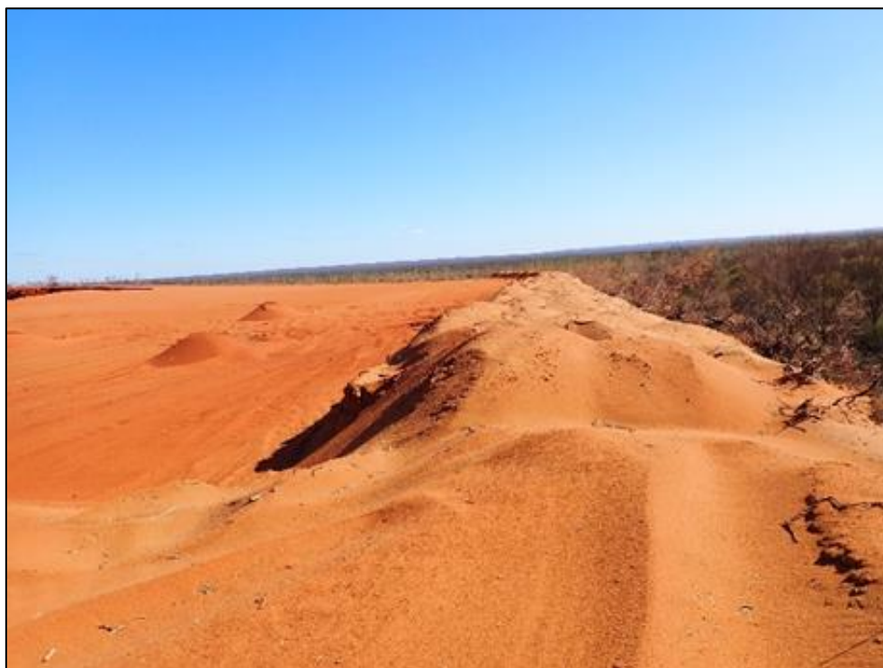
Plate 2-1 Example of Topsoil Stockpile Along Excavation Area
